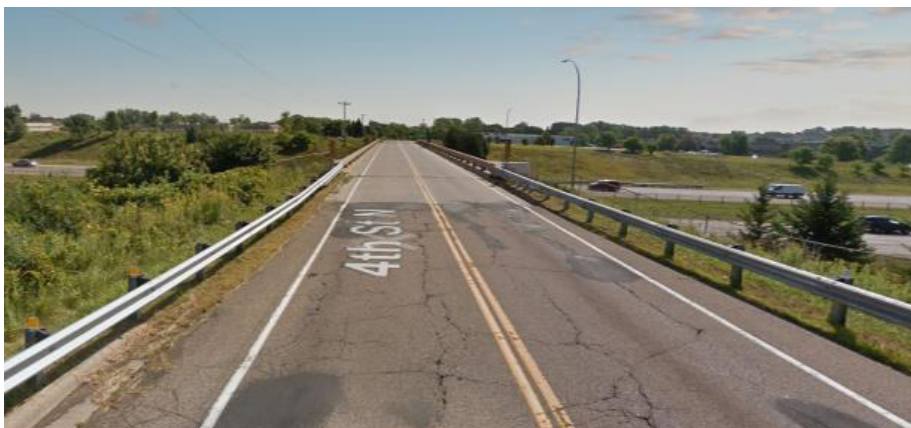
Current 4th Street Bridge
