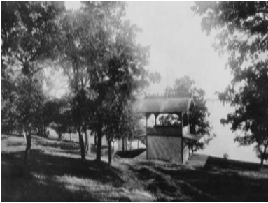
Park Structure with Lake Elmo in Background, ca. 1888
