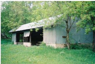
Farmstead Ruin near Eagle Point Lake
